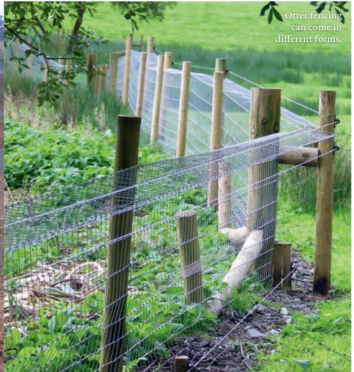
Otter fencing being erected around a new water.
